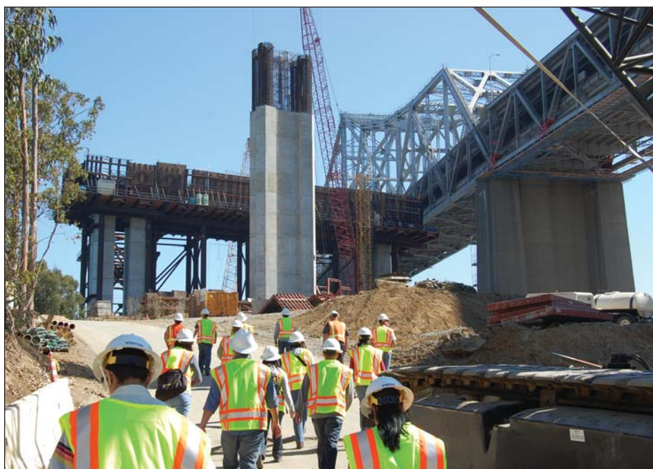
Students approach Bay Bridge project site.
