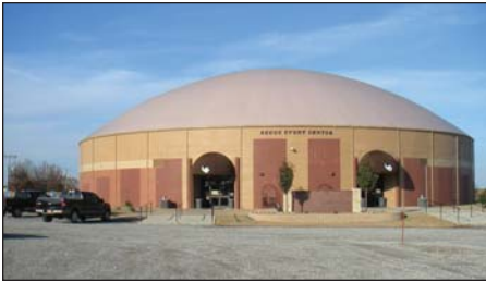
Beggs Independent School District is among eight school districts in Oklahoma that have opted for Monolithic Dome construction. Construction was recently completed on a 160-foot diameter gymnasium and event center that can double as a community disaster shelter.
