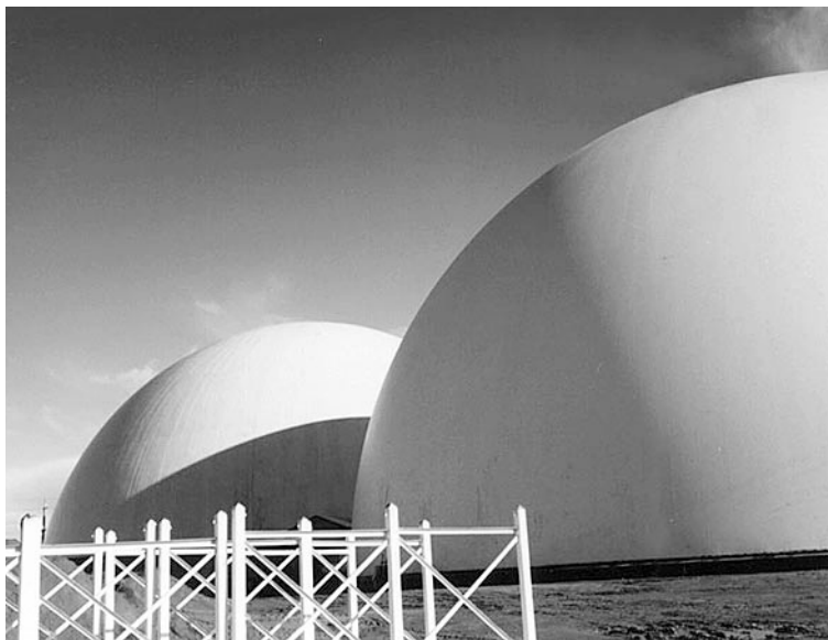
CALAMCO Cold Storage facility. Each Monolithic™ Dome is 230 feet in diameter and can store 13,000 tons of fruit — that's over 600 semi-truck loads.
