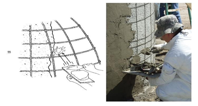
Apply first layer of concrete. Concrete can be hand applied by troweling or flipping it on, using a small mason trowel. It also can be applied with a Shotcrete pump. Be sure to place only what will stick. We now recommend application of 1/2" to 3/4" of concrete before layer of reinforcing. Then place the basalt rope after the first layer of concrete has had time to set (24 hours).
