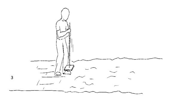
Tamp the ground with a hand tamp or mechanical equipment until it has an even, all-over firmness.
