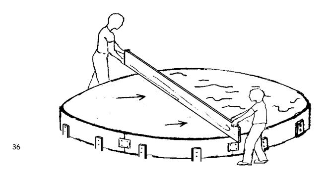
Level the concrete with a screed board as it's being poured. Excess can be moved ahead or removed. As concrete hardens, it can be troweled to a finer finish.
