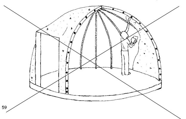
Interior plaster may require two coats. If the interior will not be subjected to water, lime can be added to those inner coats to make the troweling easier.
