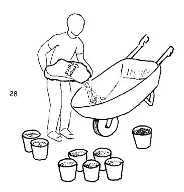
Mix the concrete in a wheelbarrow or a mixing box.
