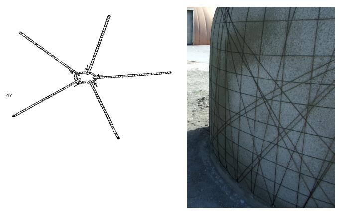
Start the rebar hanging with a few rebar tightly bent around a center ring 1.5' to 2' (45 to 60 cm) in diameter. Place the ring in the center of the Airform's top and, on the outside of the Airform, hang the starter rebar from the center ring to the perimeter. It is far better to use basalt rope or basalt rebar than steel reinforcing.
