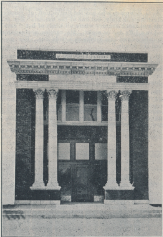
Recently completed Banking House of the Farmers State Bank, Italy, Texas
